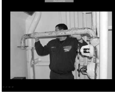
Figure 3. Photo of a “Hard” Bypass 107
